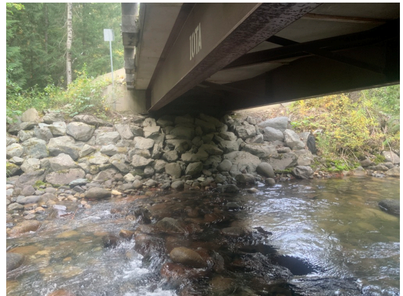
Right Bank Abutment when facing downstream
