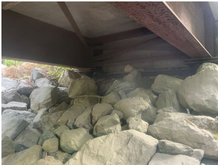
Left Bank Abutment when facing downstream
