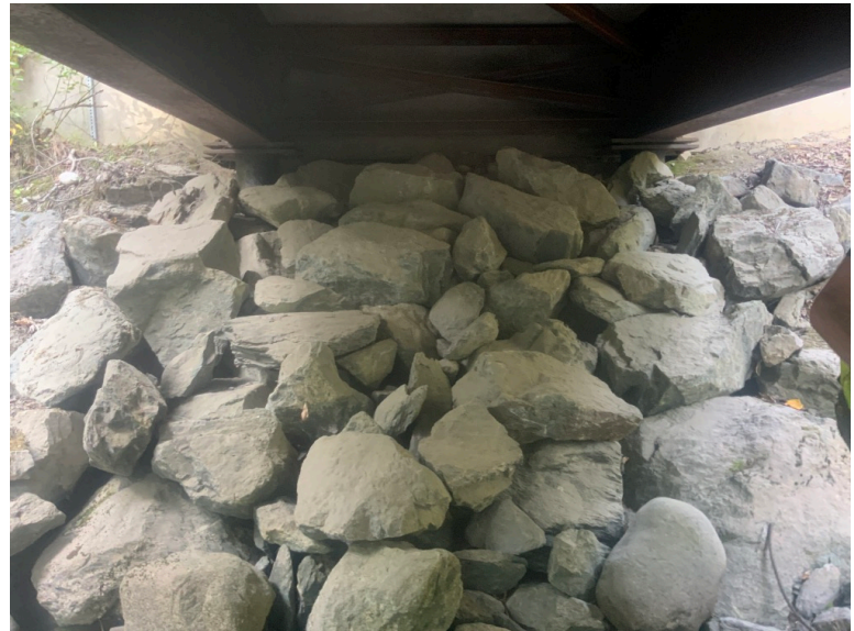
Right Bank Abutment when facing downstream
