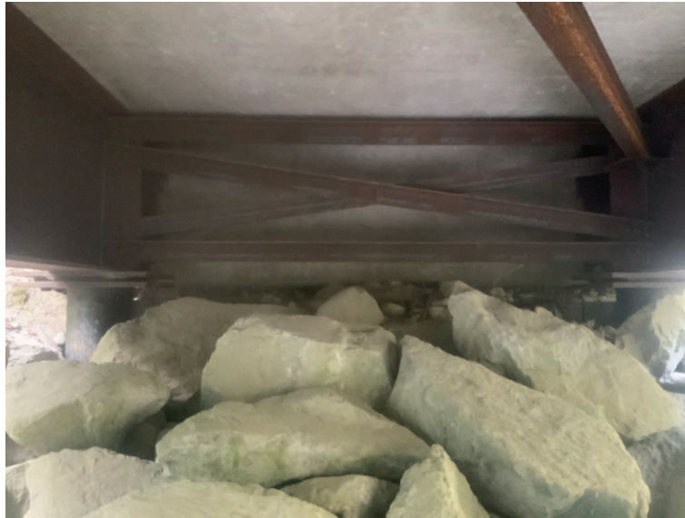
Right Bank Abutment when facing downstream
