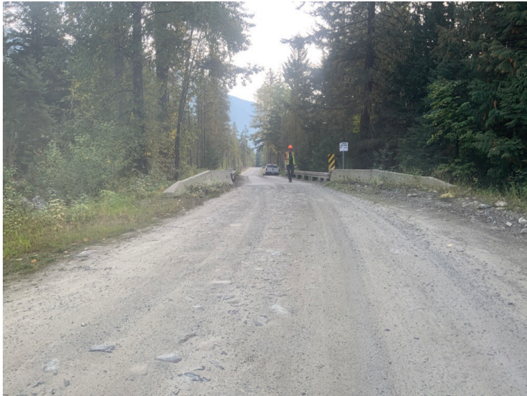
Approach from Right Bank when facing downstream
