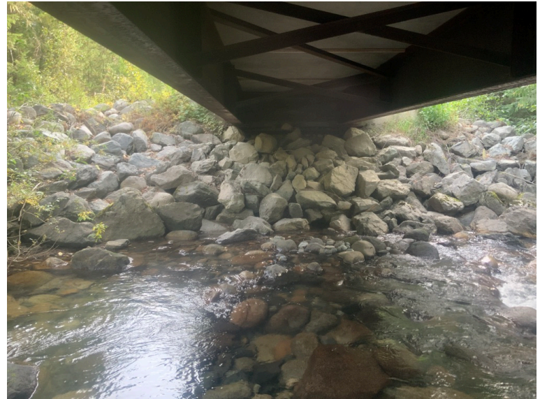
Left Bank Abutment when facing downstream
